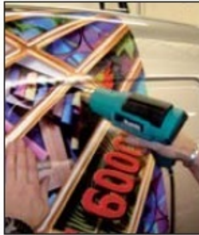
Trouble-free stretching of digitally printed film; Right-On evaporates within 3 minutes.
